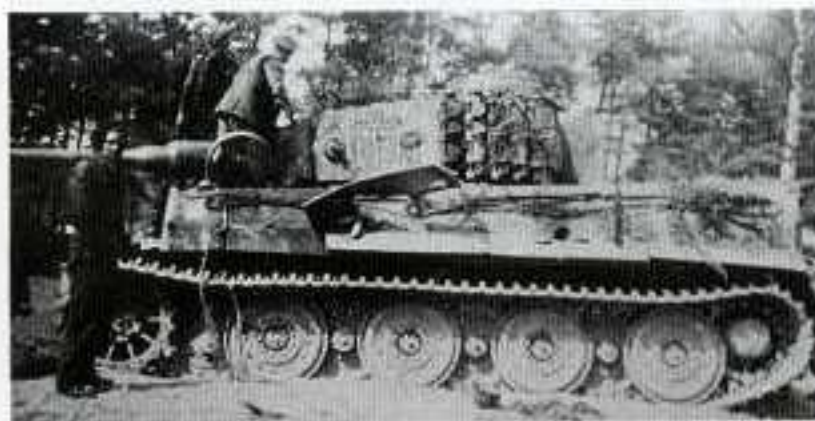
This side view of Tiger tank F01 shows the large blackened hole in the hull where Sgt. Harding's Comet tank with its 77mm main gun had surprised Unteroffizier Franzen's vehicle and destroyed it. Photo from the Giuseppa Finizie collection
