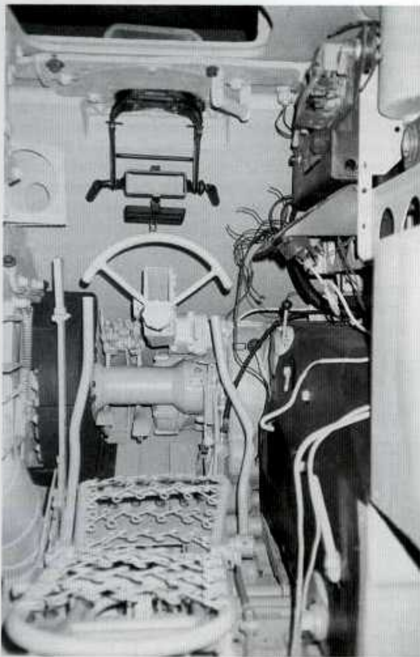
An interior view of the driver's position in the Tiger II, now on display at the US Army's Patton Museum of Cavalry and Armor located at Fort Knox, Kentucky. Unlike the box-like hull of the Tiger I, the Tiger II had a well-sloped frontal armor plate. The only hatch-down vision the Tiger II driver had was provided by a rotating periscope mounted in front of his hatch. The driver's seat was adjustable for both forward and backwards movement. The seat could also be raised or lowered, along with the steering wheel and accelerator when the driver had his head out of his hatch. The leather cushions for the driver's seat are missing from this vehicle as well as the driver's rotating periscope. Patton Museum
